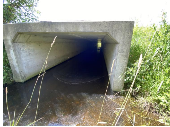
Photograph 6: Unnamed watercourse crossing at Highway 26 – looking upstream at culvert outlet
