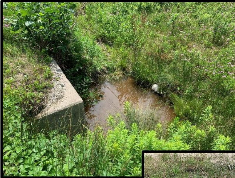
Photo 8 (left): The Bayshore Creek main exit from the property is on the south of Beachwood Road, opposite Thomas Street. After a heavy rain the area around the culvert held water but the creek channel was dry (July 29, 2021).
