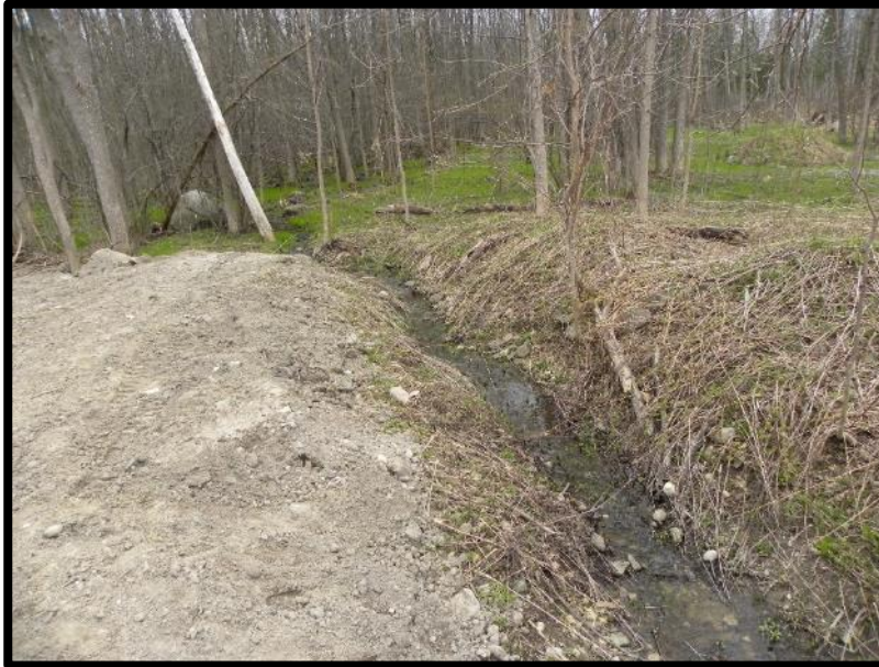
Photo 5: (left) The main exit for Bayshore Creek is a ditch on the west side of 8895 Beachwood Road. (April 19, 2021).
