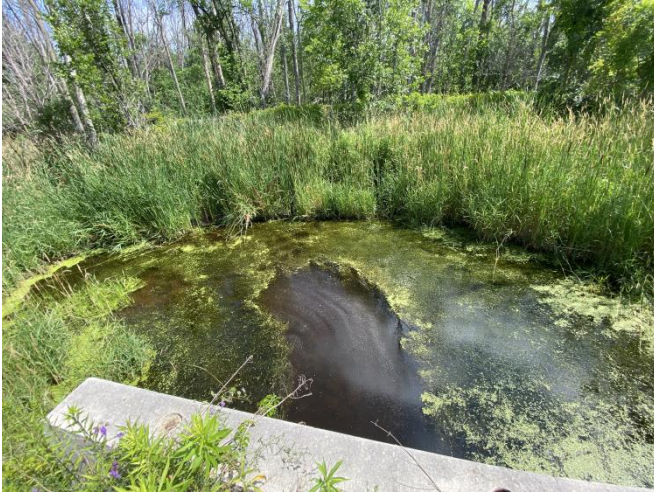
Photograph 5: SWMP outlet on north side of Highway 26
