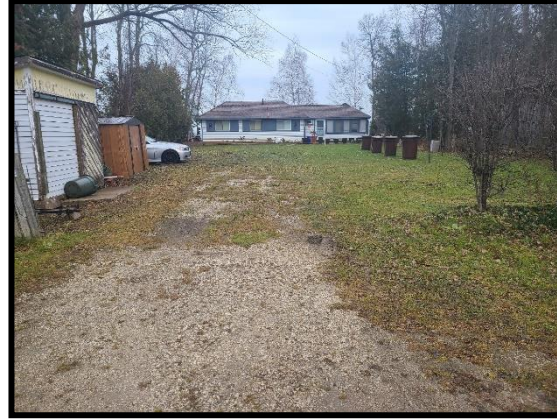
Image 18: Area of Potential (December 15, 2021; Facing Northeast)
