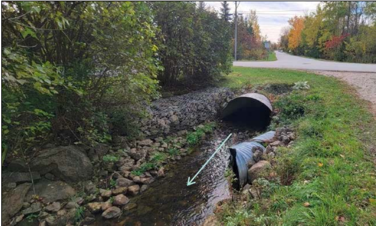
Figure 4: Watercourse crossing under Constance Boulevard at Bayswater Drive
