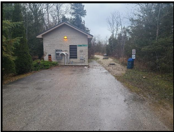
Image 3: Disturbed Lands (December 15, 2021; Facing Northwest)
