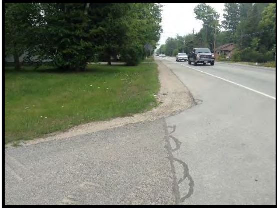
Image 17: Field Conditions (July 7, 2016; Facing Southwest)
