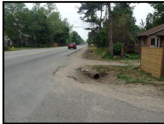
Image 4: Disturbed Lands (July 7, 2016; Facing Southwest)
