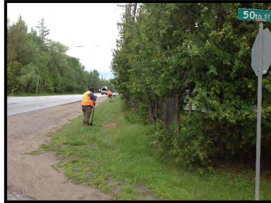
Image 24: Combination Survey to Confirm Disturbance (August 24, 2017; Facing Southwest)
