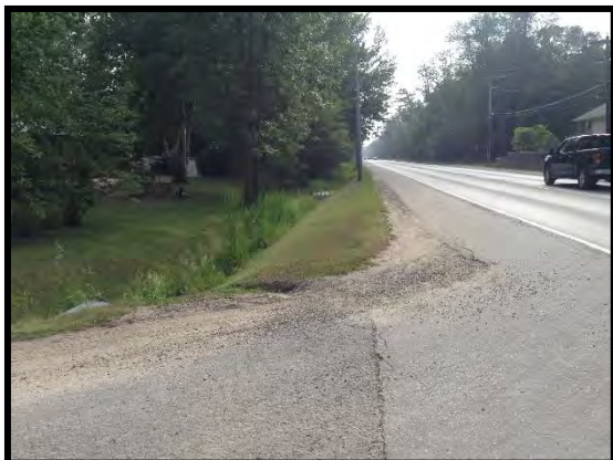
Image 15: Disturbed Lands (July 7, 2016; Facing Southwest)
