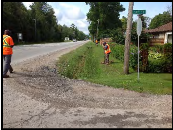
Image 29: Combination Survey to Confirm Disturbance (August 24, 2017; Facing Southwest)
