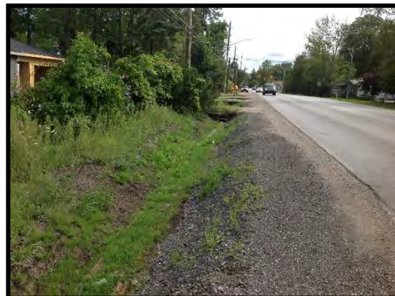
Image 28: Combination Survey to Confirm Disturbance (August 24, 2017; Facing Northeast)
