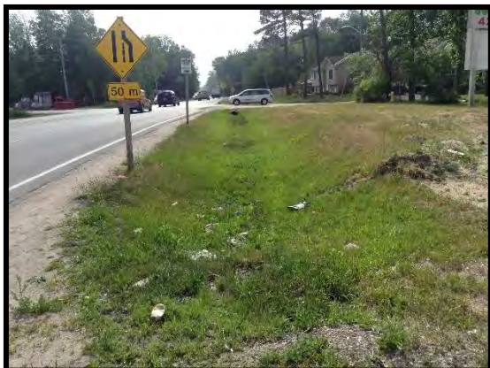
Image 21: Field Conditions (July 7, 2016; Facing Southwest)
