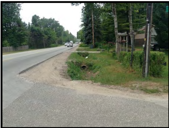
Image 3: Disturbed Lands (July 7, 2016; Facing Southwest)
