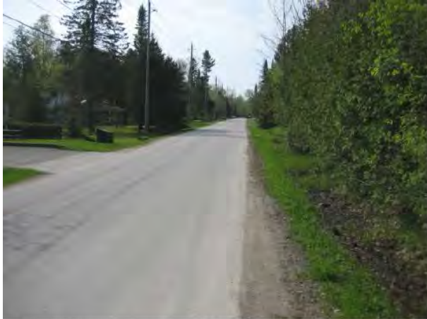
Plate 13. Northern Section of 62nd Street South (view south)
