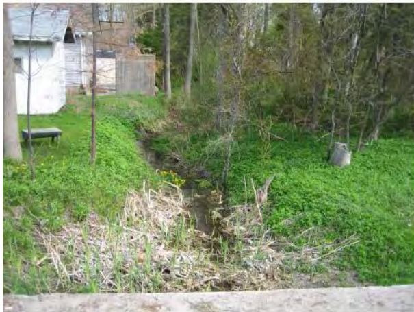
Plate 17. Watercourse and Proposed Channel Upgrades North Side of Mosley Street (view north)
