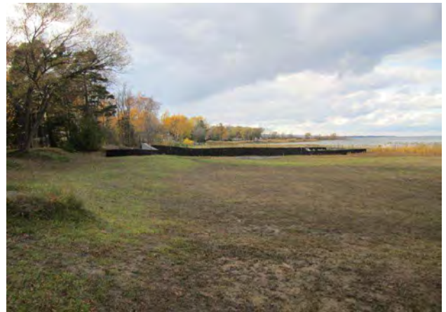
Photograph Description Overview of the 67th Street outlet
