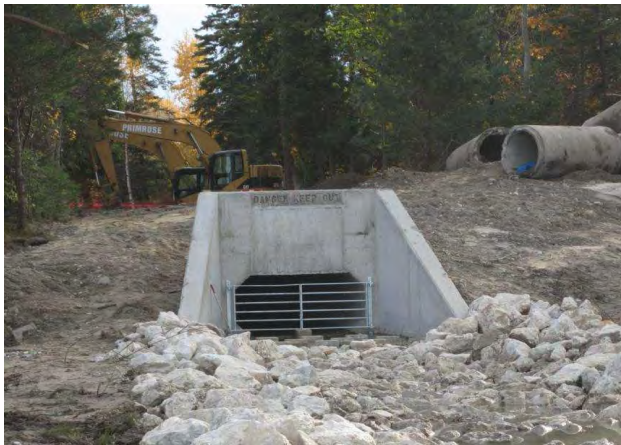
Photograph Description Outlet at 67th Street
