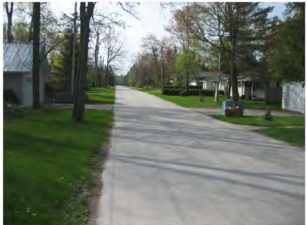
Plate 16. Northern Section of 62nd Street North (view south)
