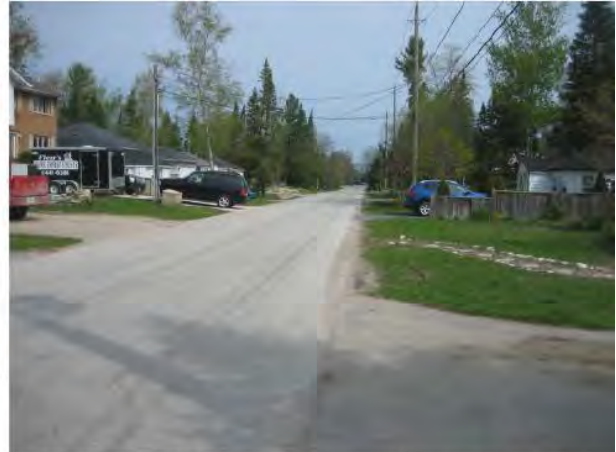
Plate 14. Central Section of 62nd Street South (view north)
