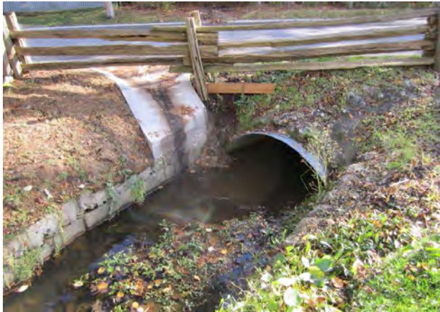
Photograph Description Outlet from culvert at Shore Lane
