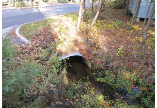
Photograph Description Inlet to culvert at Shore Lane
