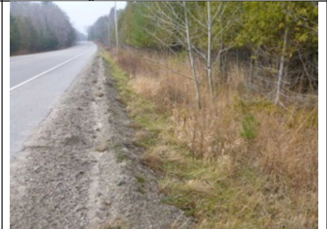
Plate 22 Steep Slope along Power Line Rd., facing Southwest
