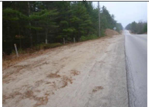
Plate 36 Shoulder of Power Line Rd., facing Northwest
