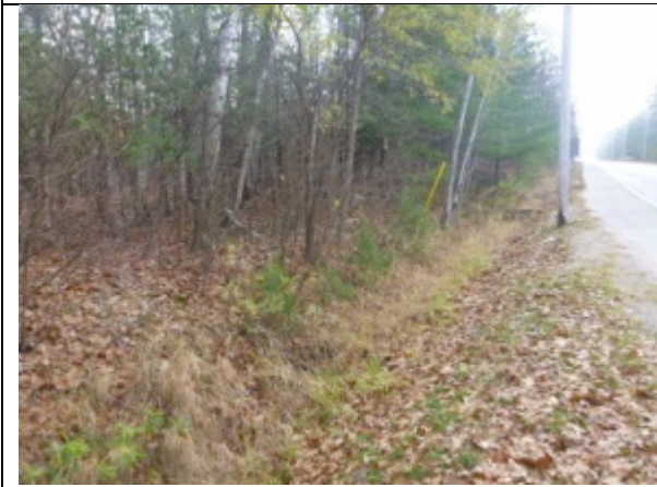
Plate 45 Drainage Ditch along Power Line Rd., facing South
