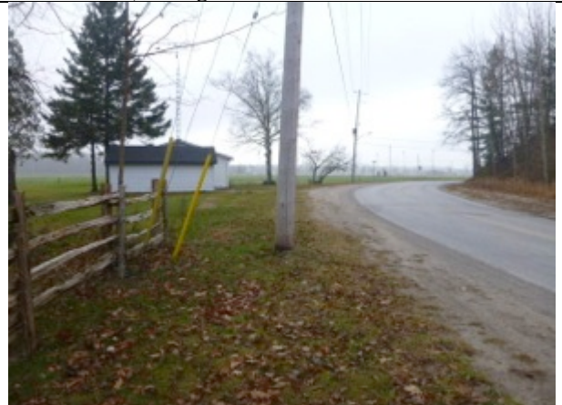
Plate 16 Shoulder of Klondike Park Rd., facing Northeast
