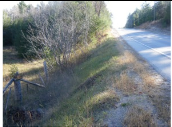
PLATE 2 TEST PIT SURVEY CONDITIONS AND STEEP SLOPE
