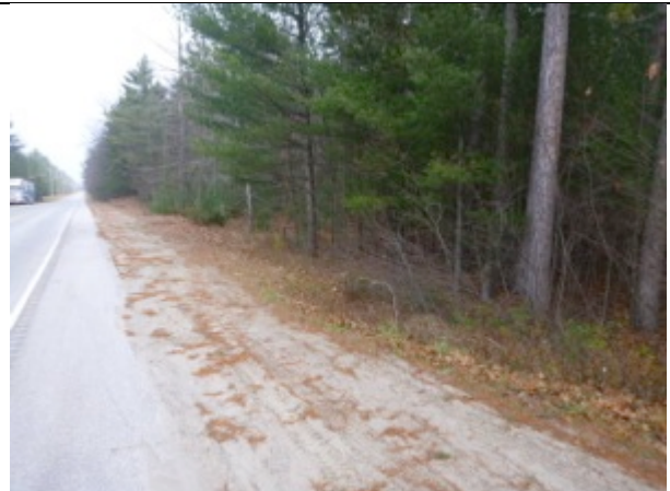
Plate 38 Shoulder of Power Line Rd., facing Northwest
