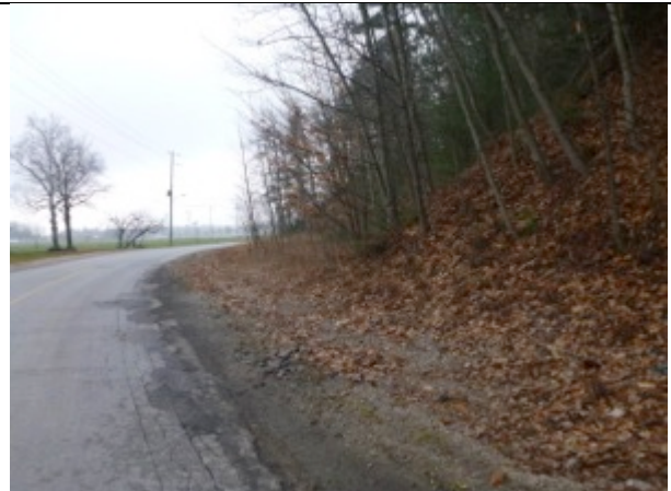
Plate 14 Steep Slope along Power Line Rd., facing Southwest
