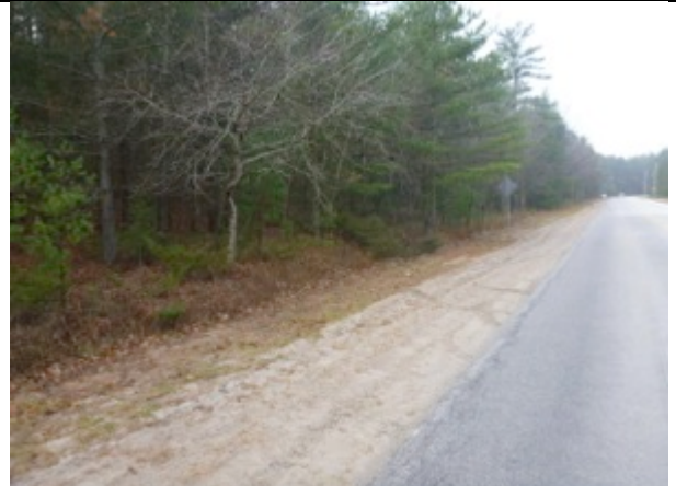
Plate 32 Shoulder of Power Line Rd., facing Northwest
