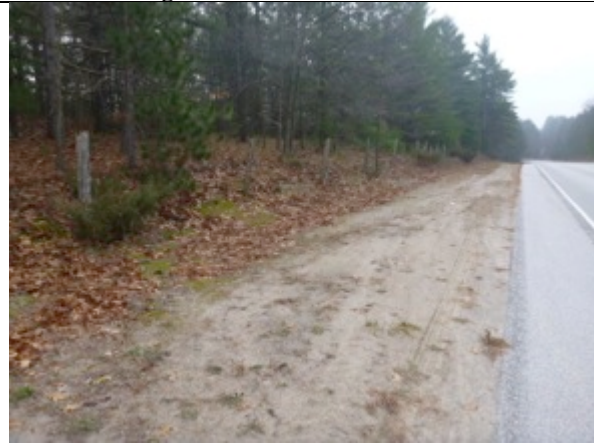
Plate 33 Shoulder of Power Line Rd., facing South
