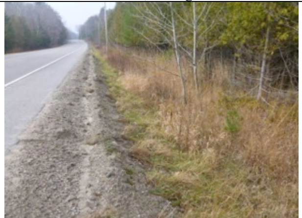
Plate 22 Steep Slope along Power Line Rd., facing Southwest
