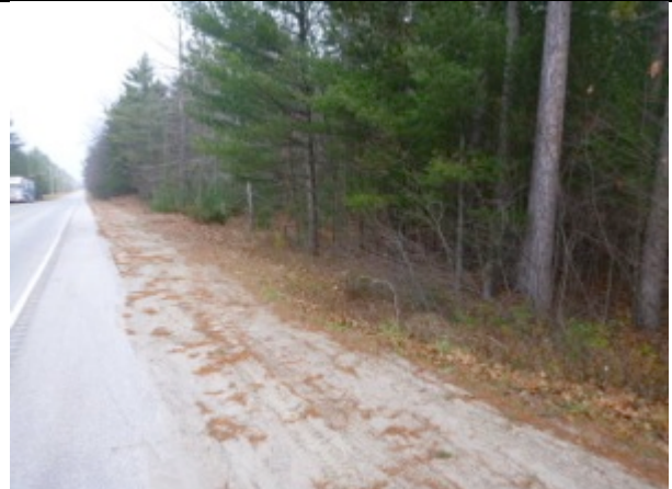
Plate 38 Shoulder of Power Line Rd., facing Northwest
