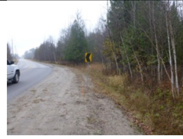
Plate 10 Steep Slope along Klondike Park Rd., facing South
