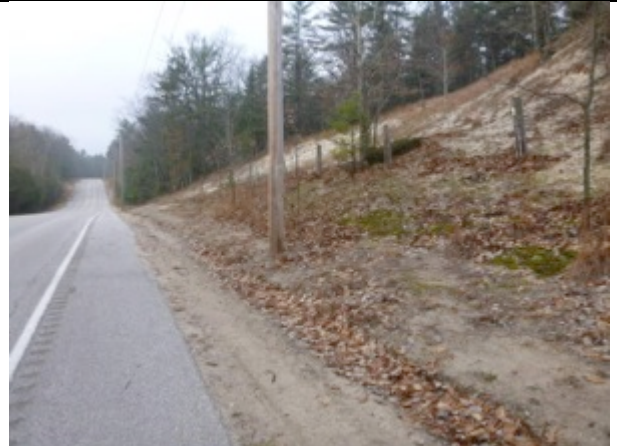
Plate 26 Steep Slope along Power Line Rd., facing Southwest
