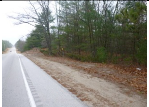
Plate 34 Shoulder of Power Line Rd., facing Northwest
