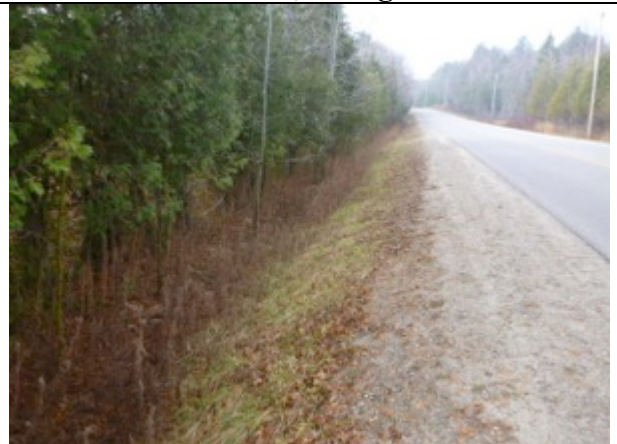
Plate 24 Steep Slope along Power Line Rd., facing Southwest
