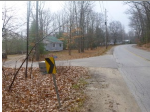
Plate 8 Shoulder of Klondike Park Rd., facing Southwest
