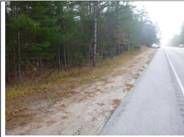
Plate 37 Shoulder of Power Line Rd., facing South
