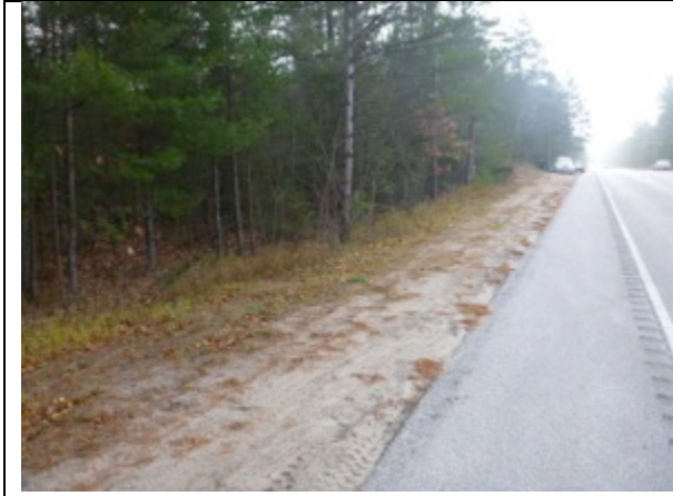
Plate 37 Shoulder of Power Line Rd., facing South
