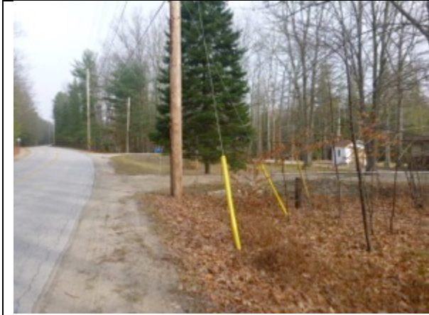
Plate 7 Shoulder of Klondike Park Rd., facing Northeast
