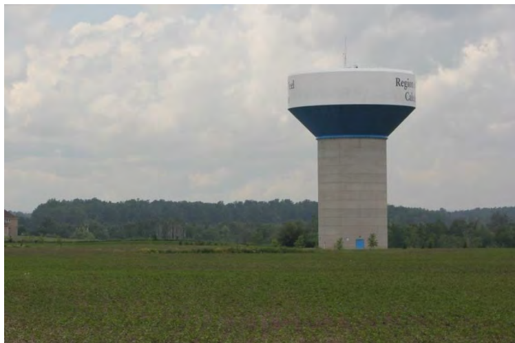
Figure 3 – Composite Elevated Water Storage
