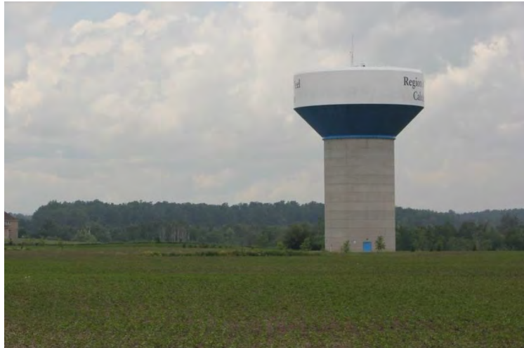
Figure 10 – Composite Elevated Water Storage
