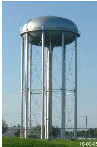
Figure 9 – Multi-Column Elevated Water Storage
