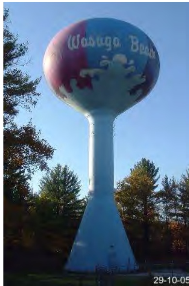
Figure 8 – Spheroid Elevated Tank located on the East End of Wasaga Beach
