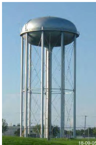
Figure 2 – Multi-Column Elevated Water Storage
