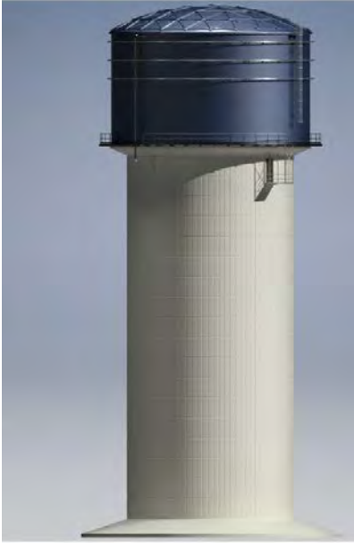
Figure 4 – Composite Glass Lined Elevated Water Storage
