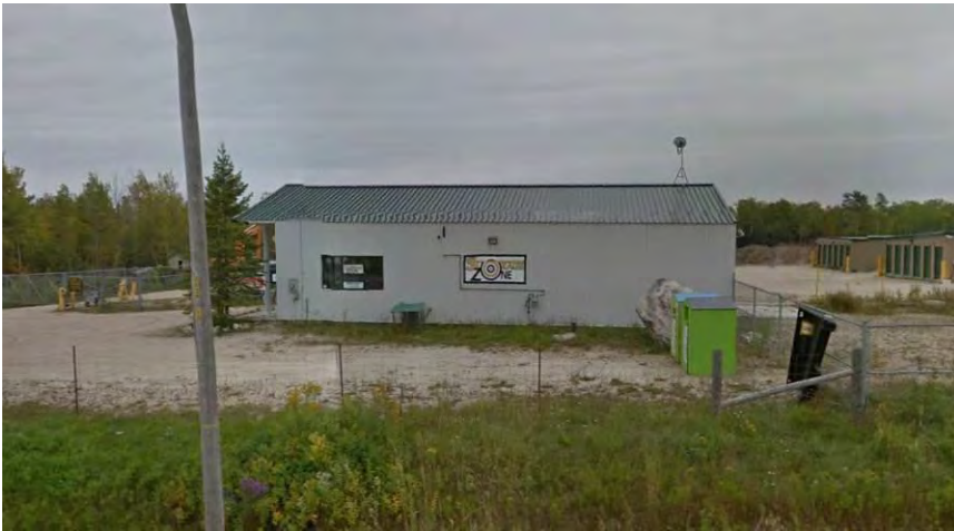
Image 1: Looking at disturbances associated with self-storage facility within Property #1.
