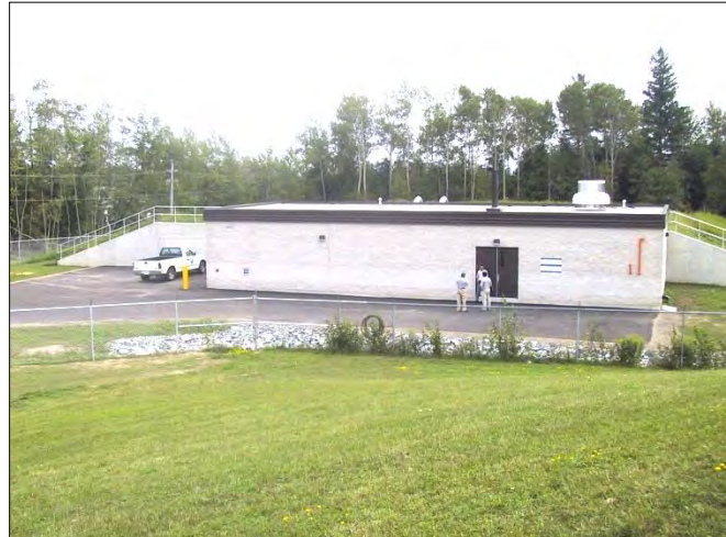
Figure 3 – Example of an In-Ground Water Reservoir (Located in Thornbury)
