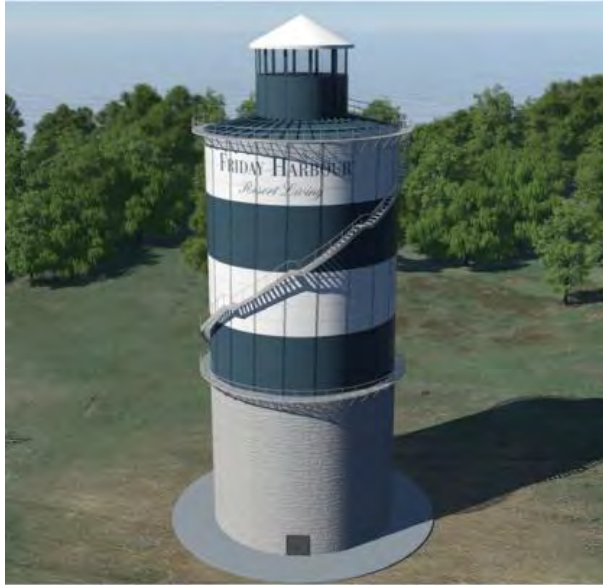
Figure 5 – Composite Glass Lined Partially Elevated Water Storage
