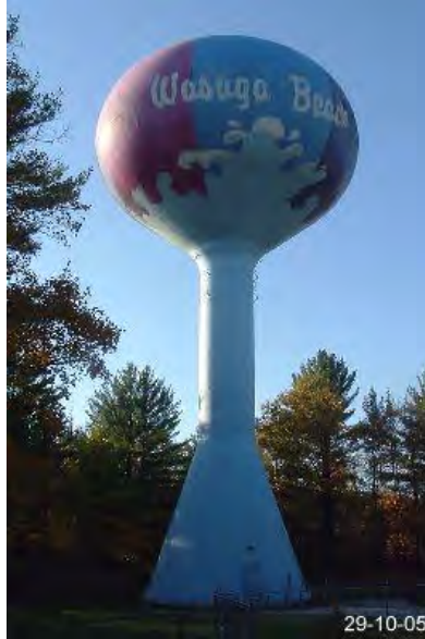
Figure 1 - Spheroid Elevated Tank located on the East End of Wasaga Beach
