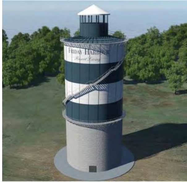
Figure 12 – Composite Glass Lined Partially Elevated Water Storage
